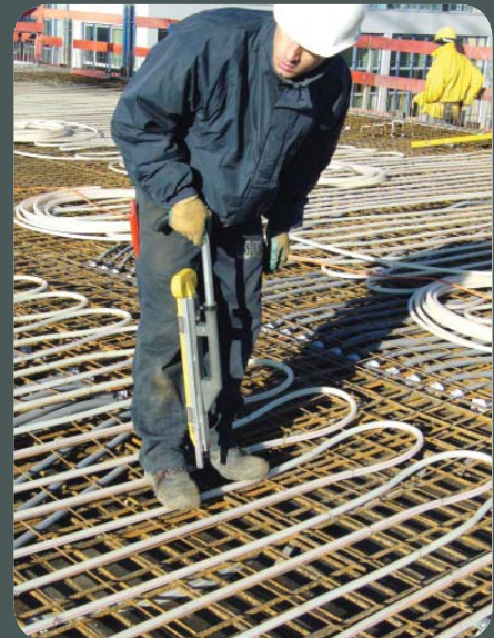
Concrete core temperature regulation
